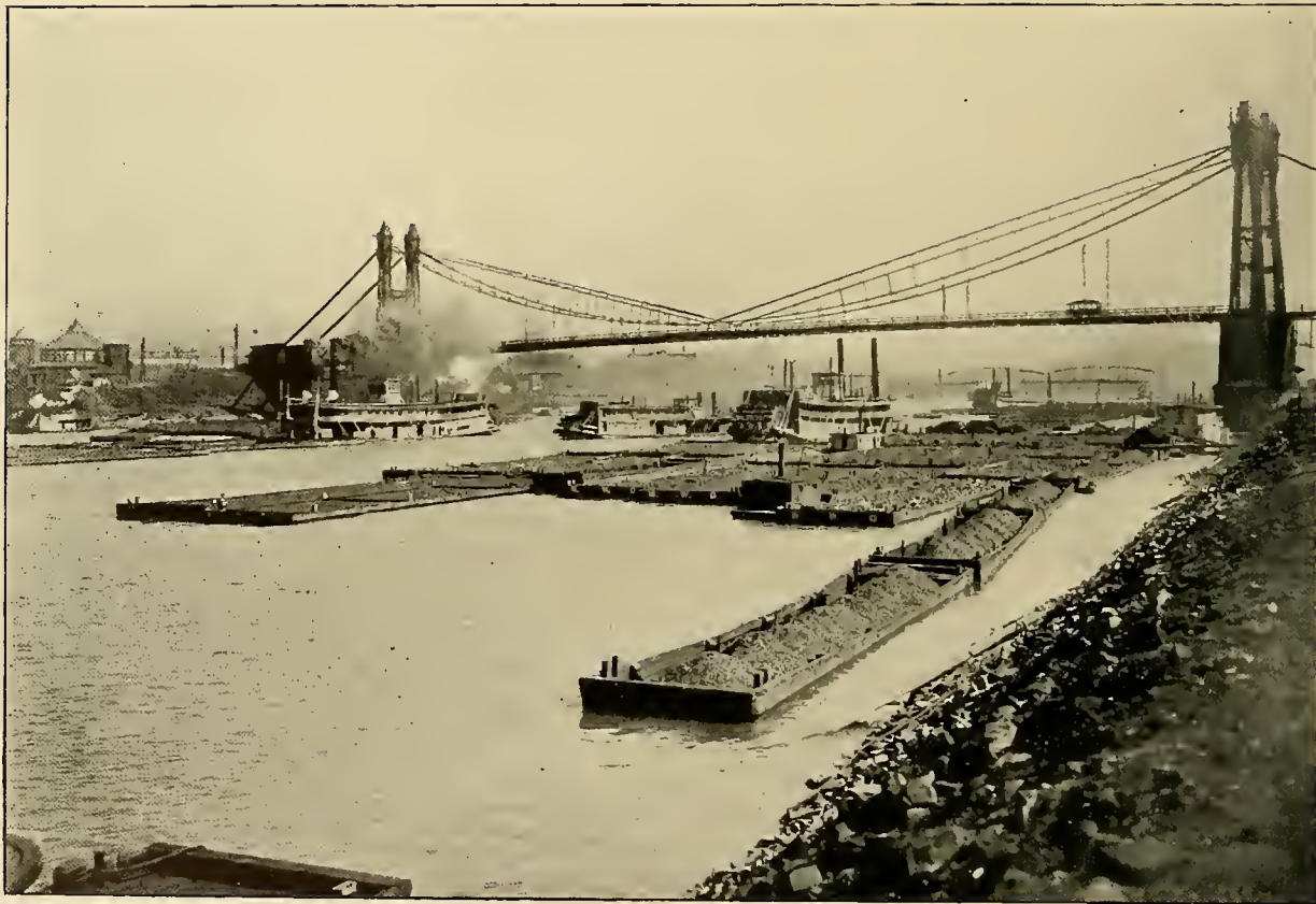
Coal Fleet below Point Bridge.
